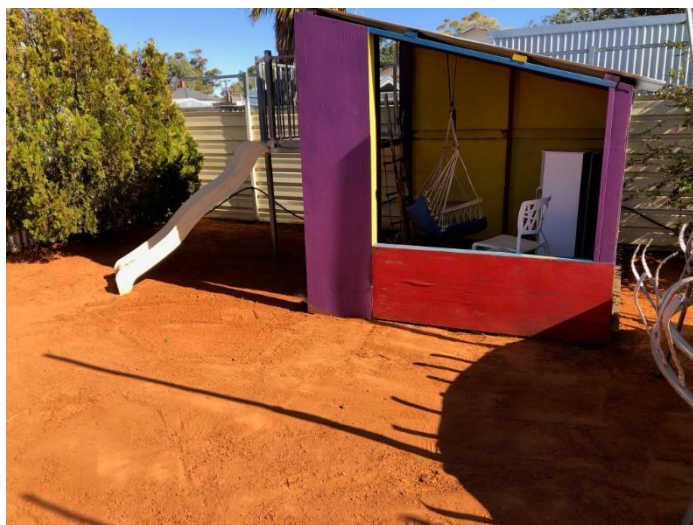
Above and below: High lead levels were detected in bare dirt and soil in the backyard of a child with elevated blood lead levels. Lead exposure risks were abated through capping and compacting the area with loam – creating a safer play environment for the child.
