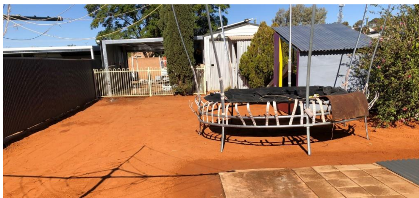
Above and below: High lead levels were detected in bare dirt and soil in the backyard of a child with elevated blood lead levels. Lead exposure risks were abated through capping and compacting the area with loam – creating a safer play environment for the child.
