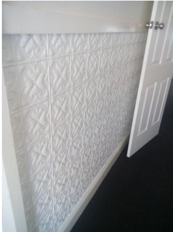
Above and below: Old, flaking and chipping lead-based paint on pressed metal walls of a hallway and on an exterior shed were identified as exposure sources for a child with elevated blood lead levels. The lead-based paint was removed safely by qualified tradespeople, the contaminated soil in and around the shed was replaced, and the surfaces were repainted.
