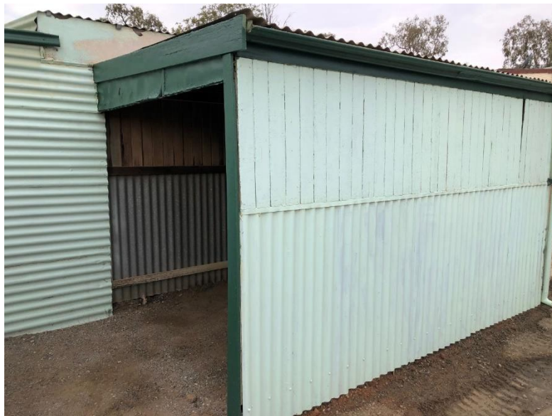
Above and below: Old, flaking and chipping lead-based paint on pressed metal walls of a hallway and on an exterior shed were identified as exposure sources for a child with elevated blood lead levels. The lead-based paint was removed safely by qualified tradespeople, the contaminated soil in and around the shed was replaced, and the surfaces were repainted.
