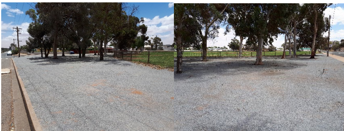
Lamb Oval footpath perimeter capped with road base
