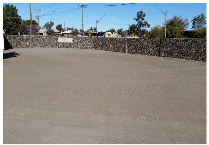
After remediation: cement-stabilised road base covers excavated area.
