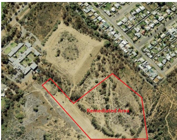
Aerial view of area remediated at University Dam.
