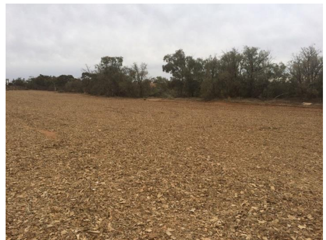
Limestone, loam and mulch were used to cover areas of bare soil following excavation works.
